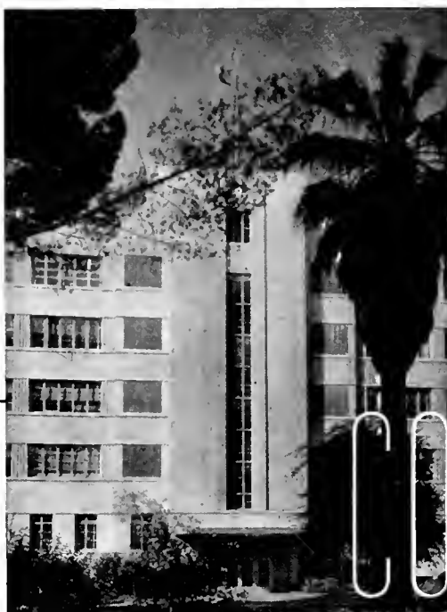
Public Works Building Twelfth and N Streets Sacramento
